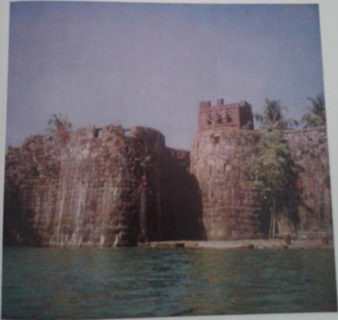
7. Main Gate of the Marine Fort, Sindkhedurg
