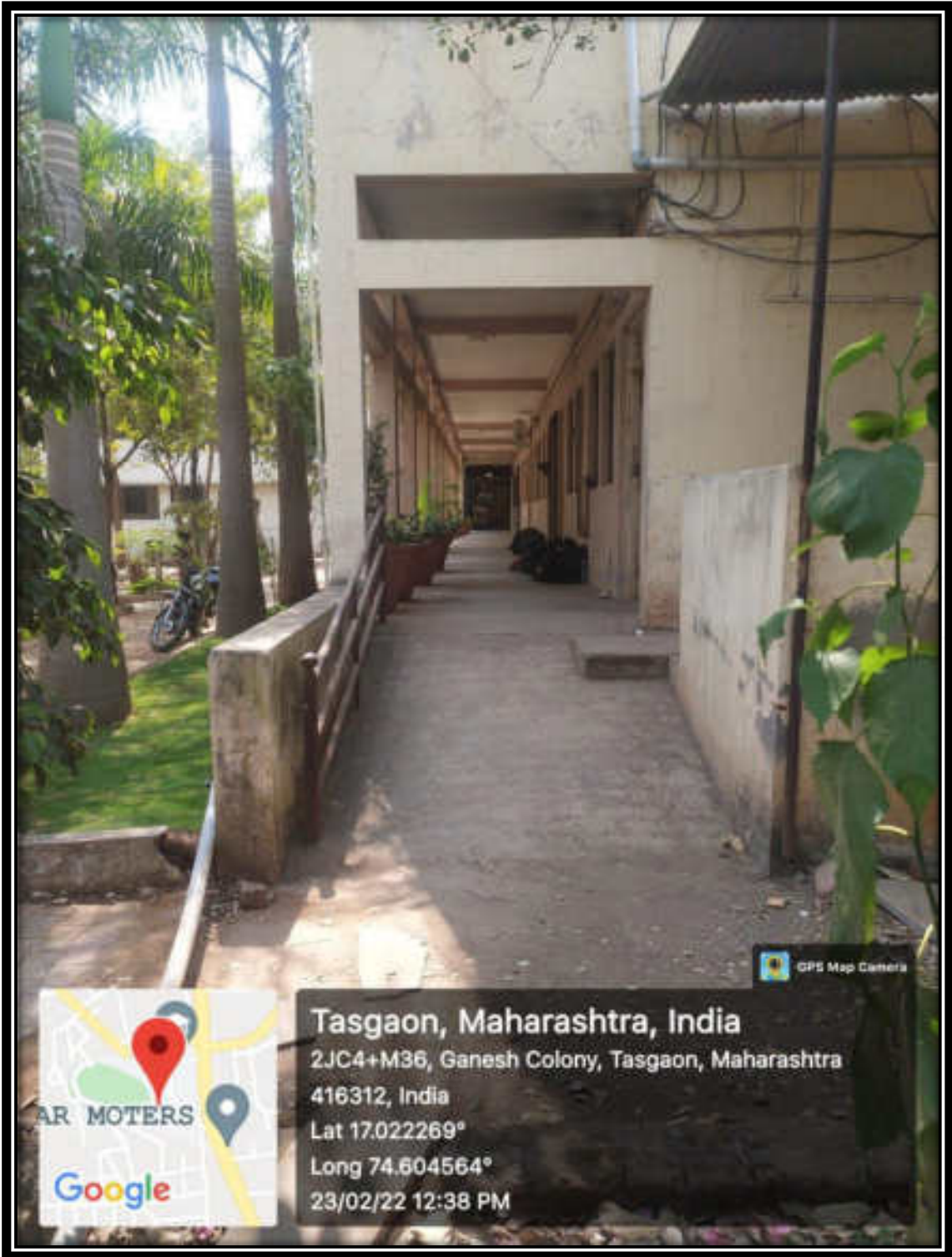
Ramp for Annex Building 01
