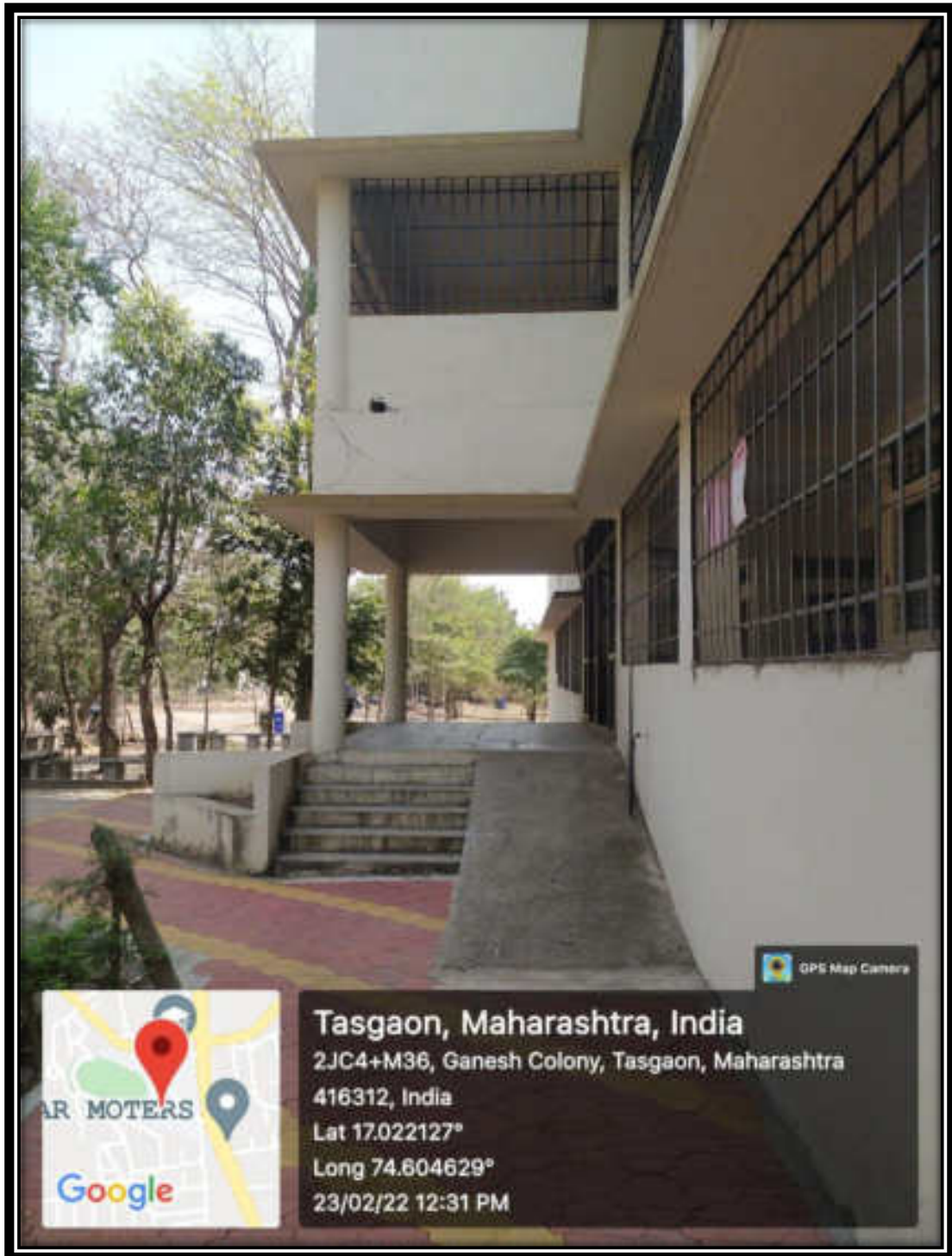
Ramp for Annex Building 02
